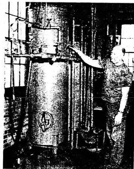
AFTER the ingredients of Skrip writing fluid have been carefully added to water in large mixing tanks, the liquid is passed through the rotating bowl of a high-speed centrifuge, which develops a force thousands of times greater than gravity. Solid impurities which may have been in the raw materials are deposited on the walls of this bowl, leaving a purified liquid. The principle is the same as that of familiar cream separators. Only about a handful of material is removed from each 10,000 gallons, but this would be enough to affect the writing qualities. In this picture Mickey Finley is removing a sample from the centrifuge to be sent to the lab for testing.
